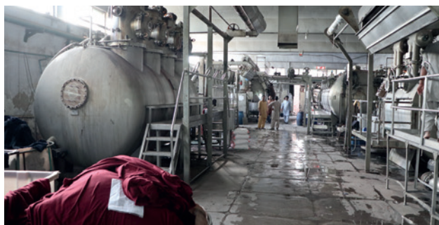
Figure 2: Water use in textile finishing (© FIW e.V., Aachen).
