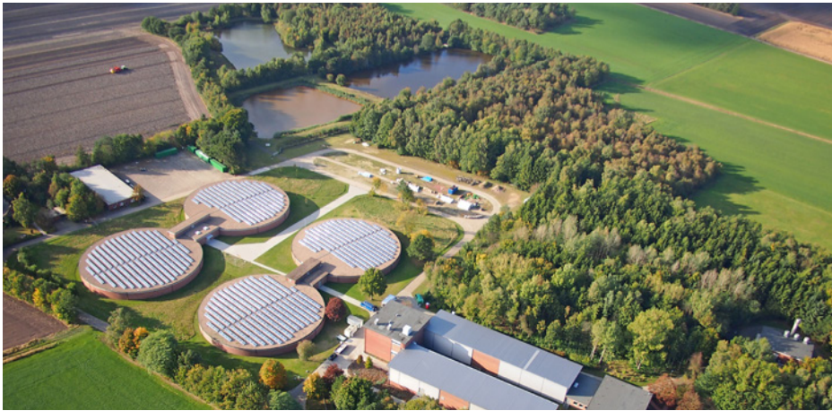
Figure 1: Waterworks in the county of Oldenburg, Germany. The regional water supplier and farmers cooperate on a voluntary basis to reduce nitrate in groundwater (© OÖWW).
