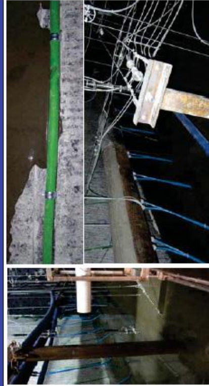
Concreting of the Drift Seal (484 m³ - fresh in fresh, Construction Time: 20 h - 15./16. Dez. 2010)
