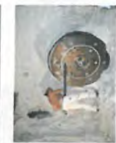
Crushed salt backfill
