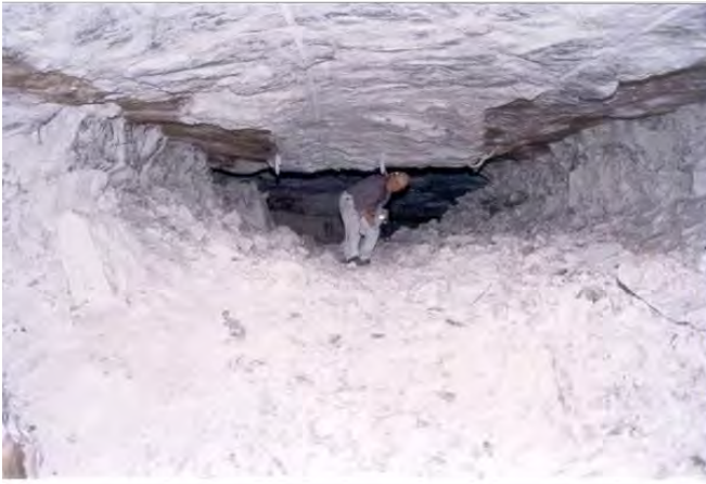
Figure 4-2. Mine collapse following a rock burst (Popp 2016), left: a photo in the collapsed region, right: measured surface subsidence compared against simulation predictions at the time of the rock burst.
