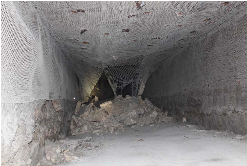
Figure 6-1. Roof fall in WIPP Panel 4 access drift (WIPP Update Oct 3, 2016).
