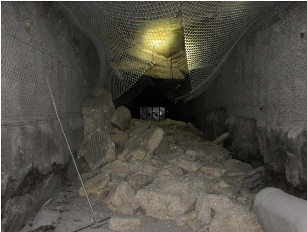
Figure 6-2. Roof fall in WIPP Panel 3 access drift (WIPP Update Oct 5, 2016).
