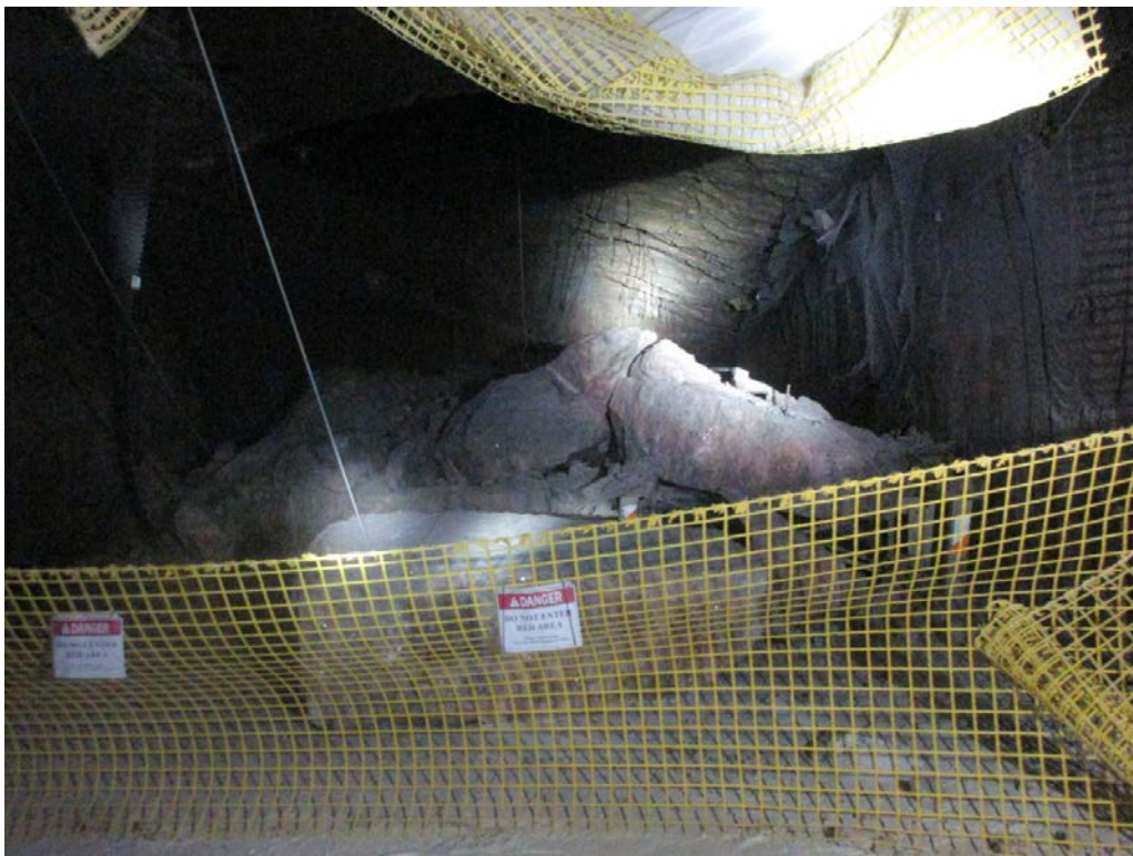
Figure 6-3. Roof fall in WIPP Panel 7 Room 4 (WIPP Update Nov 4, 2016).
