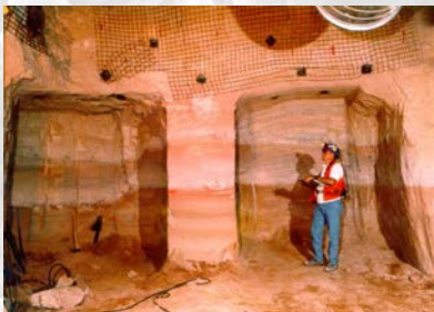
YM-19894 1 METER BLOCK EXCAVATION ACTIVITIES AT BUSTED BUTTE.
