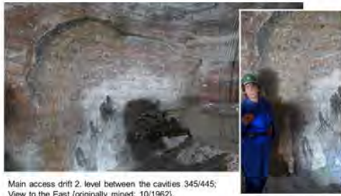
Main access drift 2. level between the cavities 345/445; View to the East (originally mined: 10/1962).
