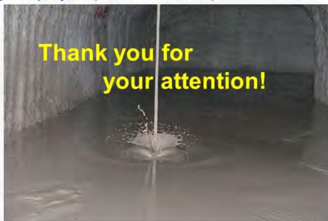
Casting of MgO-Concrete
