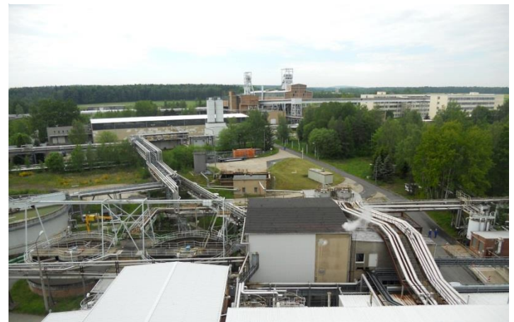
waste water treatment
