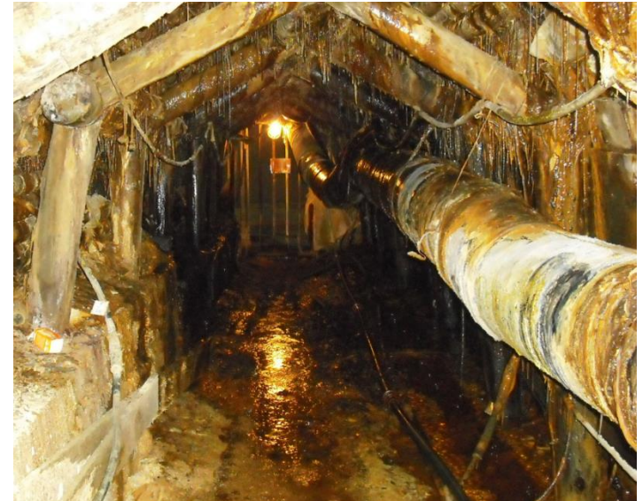
underground before flooding
